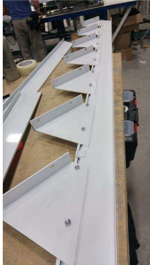
4) Assembly of stair supports on the S100 stringer
